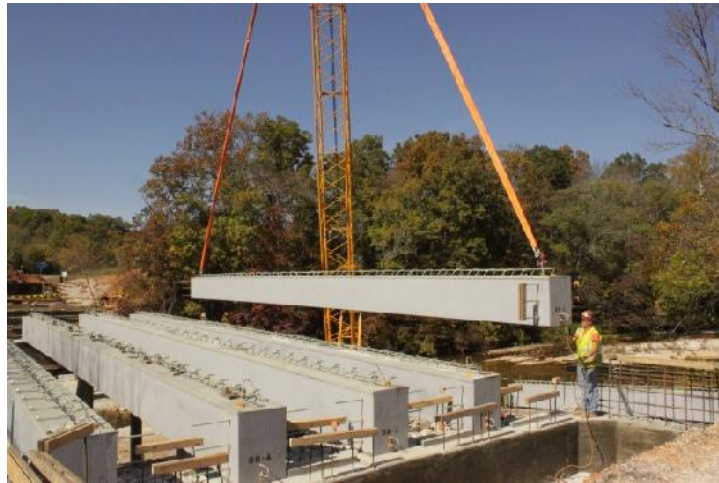
Fig. 2. B0439, HCB Erection Process
