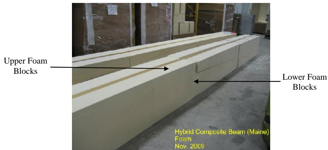
Fig. A-3. Cut and Preparation of the foam blocks
