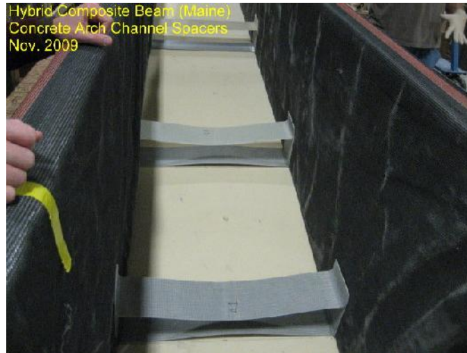
Fig. A-5. Spacer's installation
