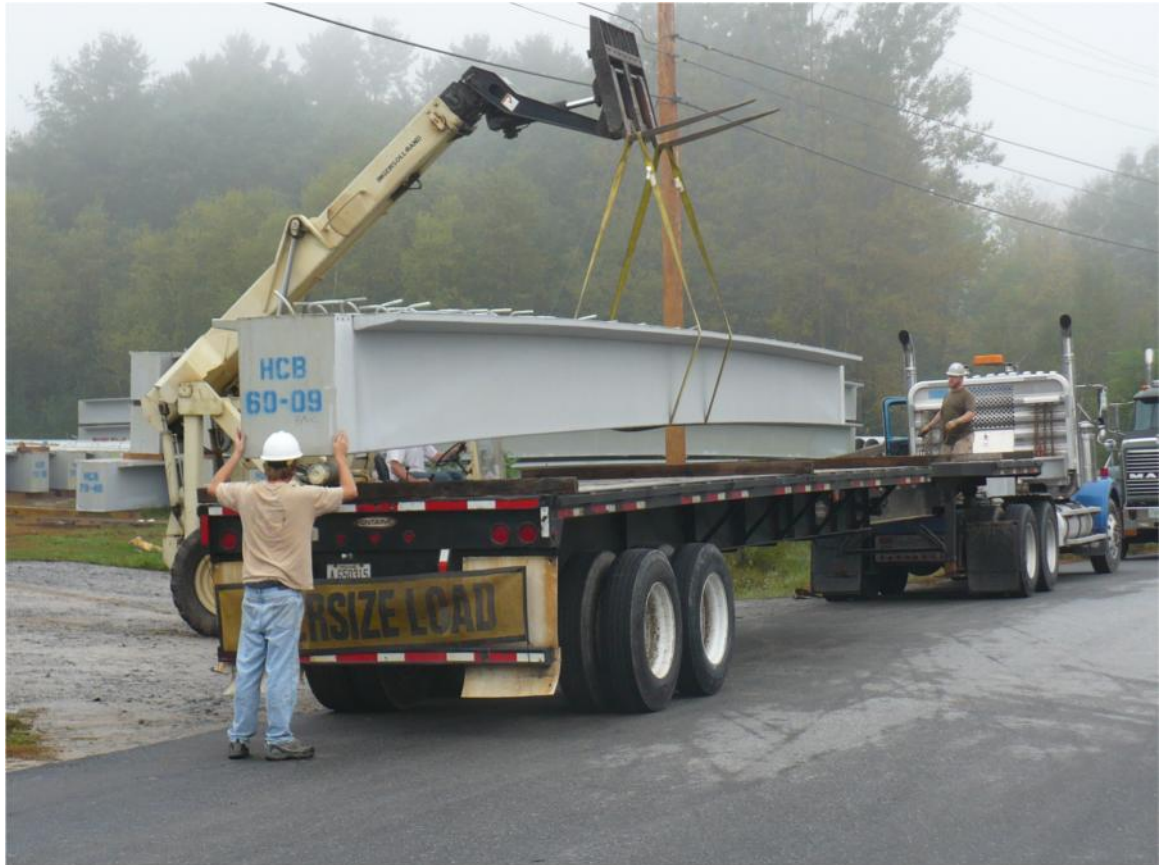
Figure 1.7. Loading of HCBs via small crane
